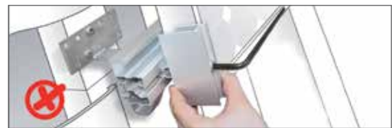
Do not use extended Allen keys!
